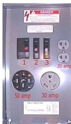
Your RV will be either a 30-Amp rig or a 50-Amp rig. How do you know? The simplest method is to check the plug on your power cord. If it is a large plug with three prongs, it is 30 amps. If it is a large plug with four prongs, it is 50 amps.
